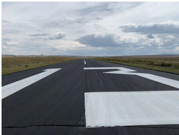
Looking south down runway 13. Highway 69 is just visible on the right.
