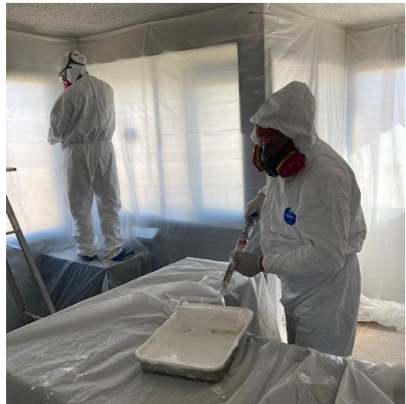
Becky Kinder and Gary Baker work on asbestos mitigation. Photo by Chris Dunmall
