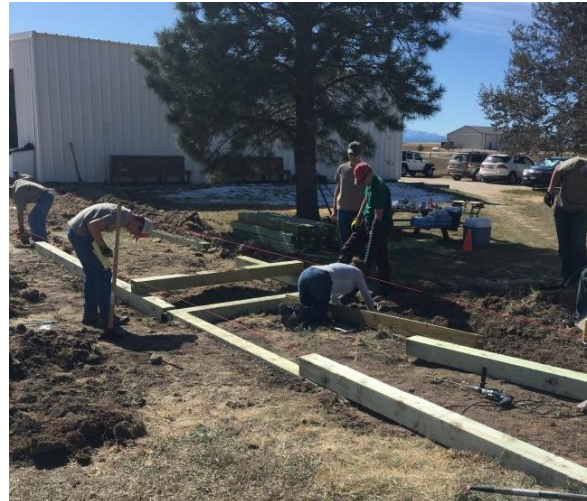
Henry Paluch and crew start work on the new walkway.
