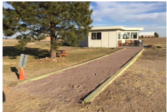
Almost done! Rails and detail work to come.
