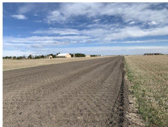
Rebuilding the runway starts with grinding up the old one.
