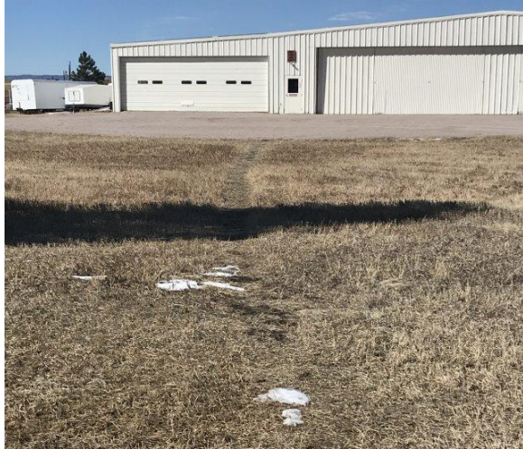
The Buildings and Grounds manager asks you to walk to the left or the right of the current path to the 3 rd Hangar. As you can see, the path is creating quite a rut.
