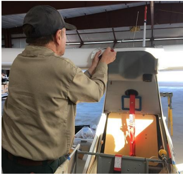
Doug installs the top window.
