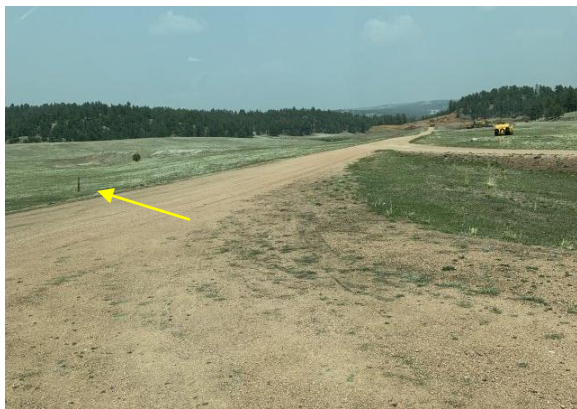
Looking NE at the intersection. See stake at the left side of picture.
