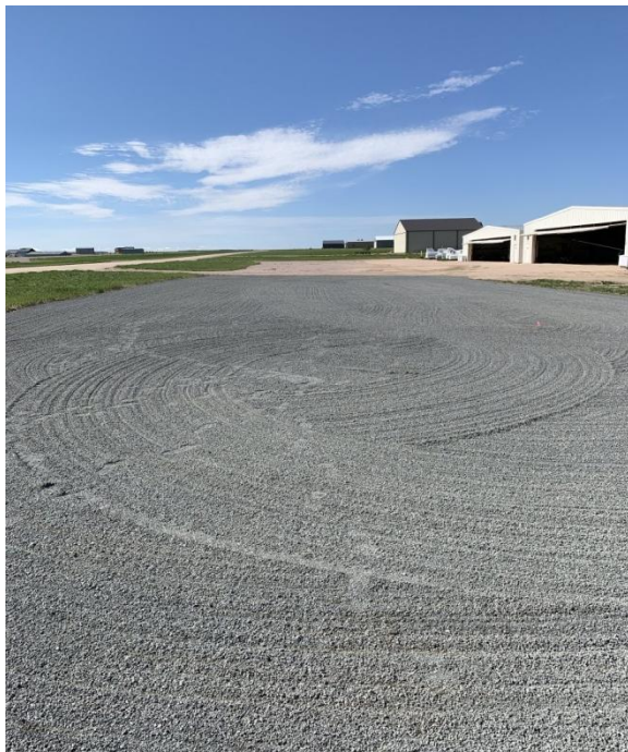
New assembly area
