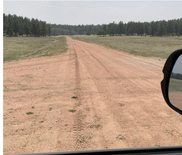
At intersection, looking SW along RWY 22. Slight slope uphill at the very end. Did not see stakes in this section. Note dropoff on the left as we look SW.
