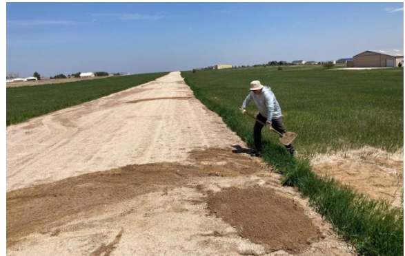
Wojtek Tomanek fills in some of the ruts. Photo by Roland Laning
