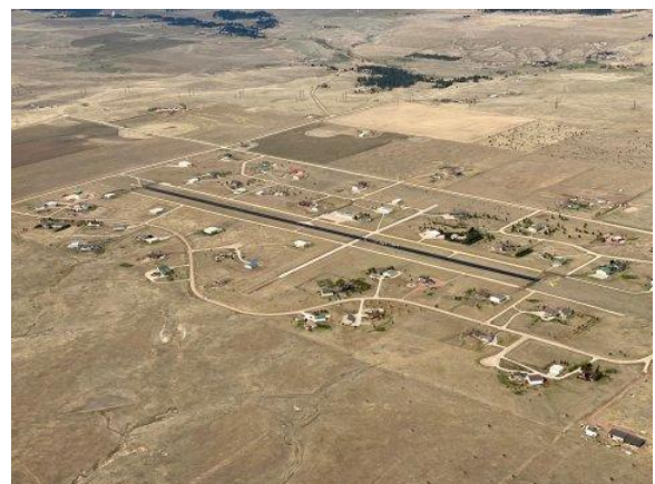
Stan Bissell captured the runway paving from the air.
