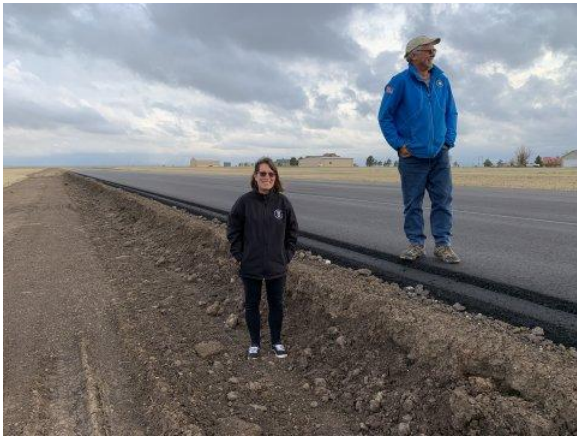
Bit of a dropoff on the runway edge, soon to be mitigated
