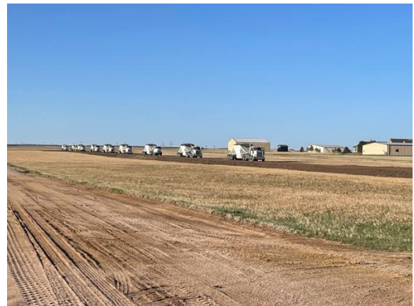
"Let the paving begin!" Photo by John Gillis
