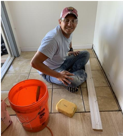
Brandon works on the new tile entryway.
