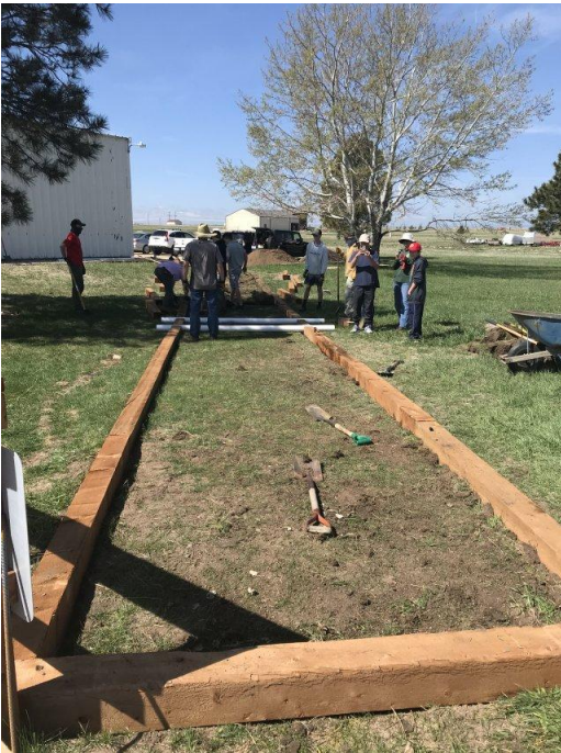
Work begins on the project. Photo by Becky Kinder
