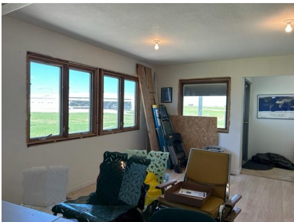
More pictures of the windows installed by Frank, Gary, and Chris
