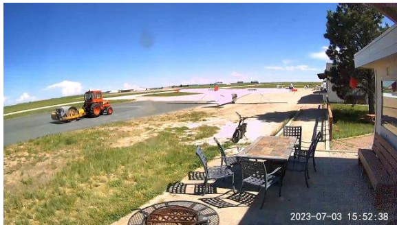
Dave Allen rolling the new assembly ramp
