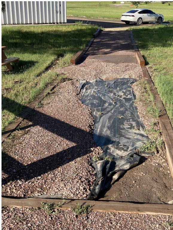
The main walkway took heavy damage from the June storms.
