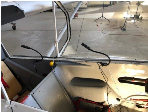
Big thanks to Doug Curry and Dave Rolley for installing boom mikes in 840!
