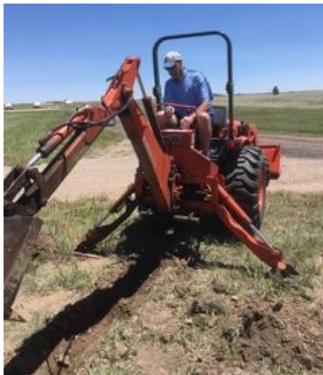
Bif Huss mans the digger (photo by John Mann)
