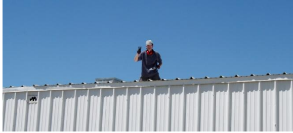
Steve Johnson working on the roof of Hangar 3
