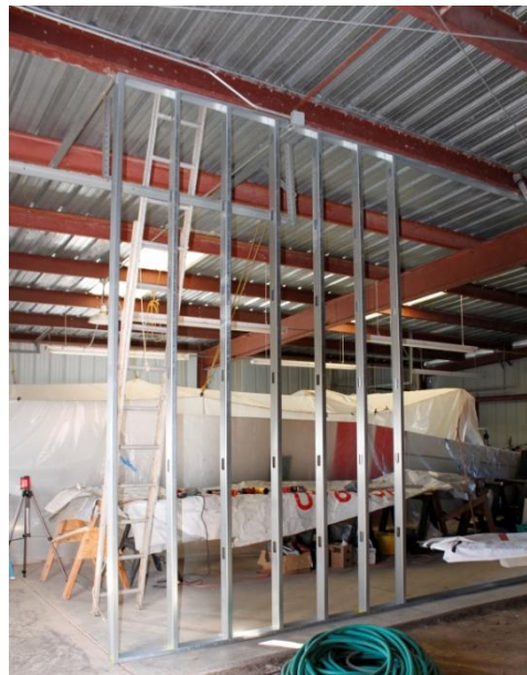
Work begins to enclose the shop area in Hangar 3.
