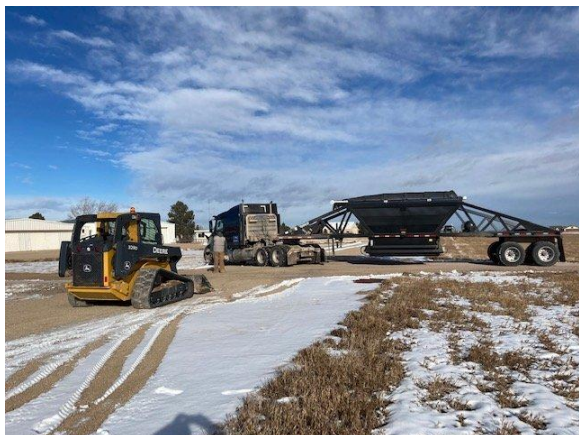
Work on the ramp. Photo by Chris Dunmall.
