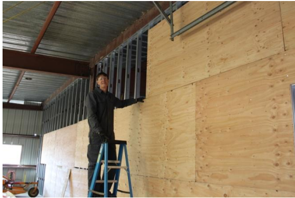
Steve Johnson installing the new shop wall
