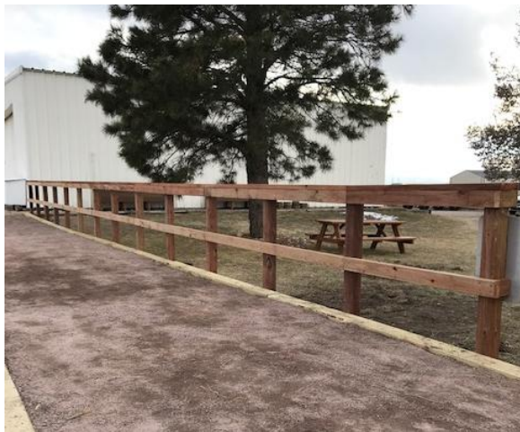
New walkway. Photo by Raul Boerner.
