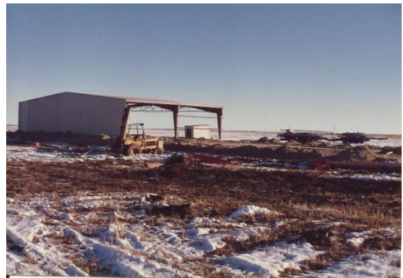
Hangars Start to Go Up
