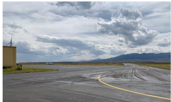
The ramp at Westcliffe
